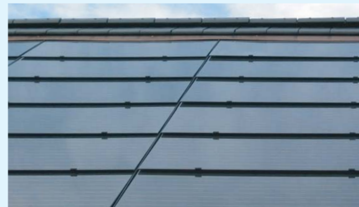
The frameless MegaSlate® solar laminates are shingled like traditional roof tiles.
